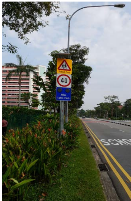
Fig 1. “40 km/h When Lights Flash” sign installed at Northland Primary School
